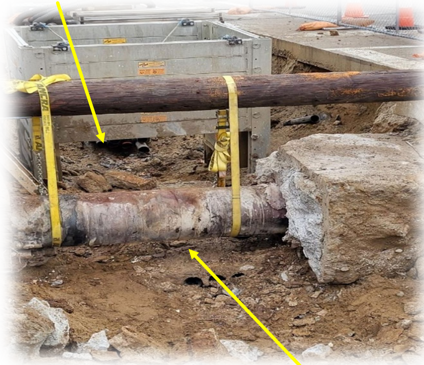
Broken duct
